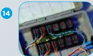
14 Commoning Blocks for Distribution in IW
